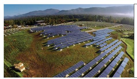
Green Mountain Power and the City of Rutland have installed the Stafford Hill plant (Left). This is a solar and battery system that can disconnect from the grid and supply critical power to an emergency shelter during long outages.
